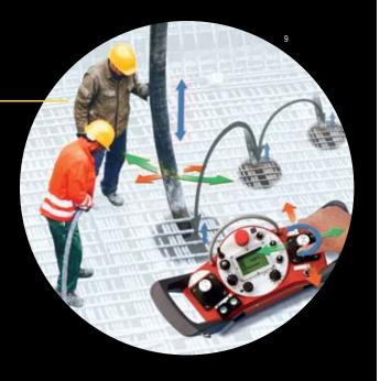
In addition to putting the power of EBC at your fingertips, the OneTouch controller provides accuracy without the need to switch to different boom arms. On five-section booms the positions of the "A" and "B" arms can be locked. Once the position has been saved, the arms remain in their position, regardless of how the other arms are moved. A preferred position can be set for the last arm. This position is maintained during concrete placement.
